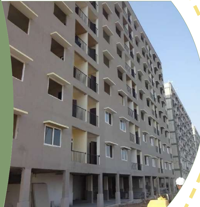
Photograph showcasing light-colored exteriors with windows and inset balconies for shading to reduce heat gain and sufficient daylighting
