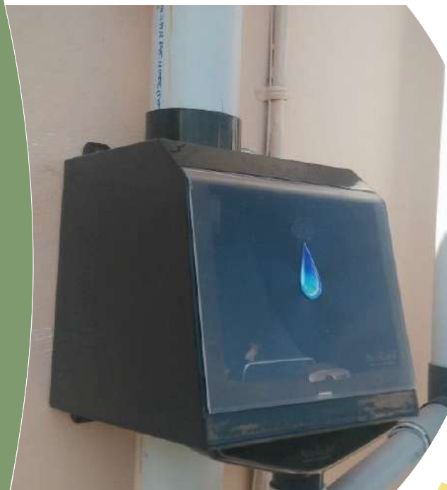
External device for mechanical rain water filtration
