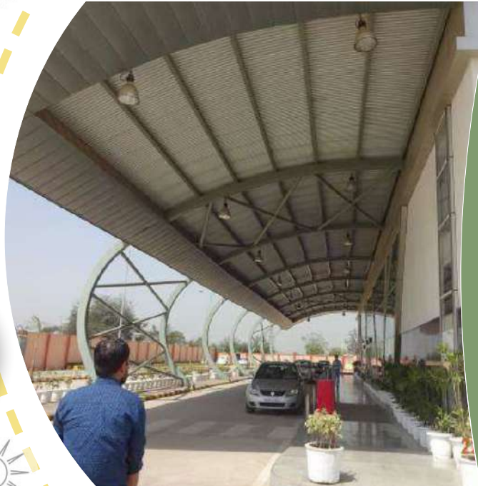
Image showing the large overhangs for shading of building facade & entrance
