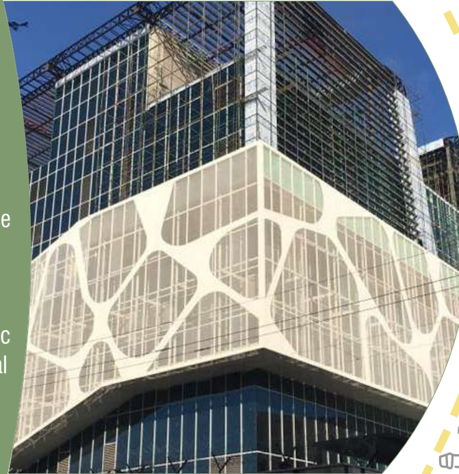
Image showcasing the shading devices integrated into the building façade, effectively minimizing direct heat gain and enhancing energy efficiency
