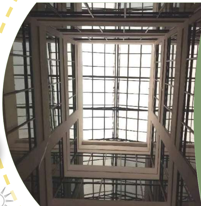
Image showcasing a polycarbonate-covered courtyard designed to maximize natural daylighting within the building
