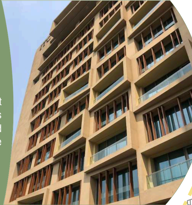
Close-up image of the facade highlighting diverse shading strategies tailored to different orientations
