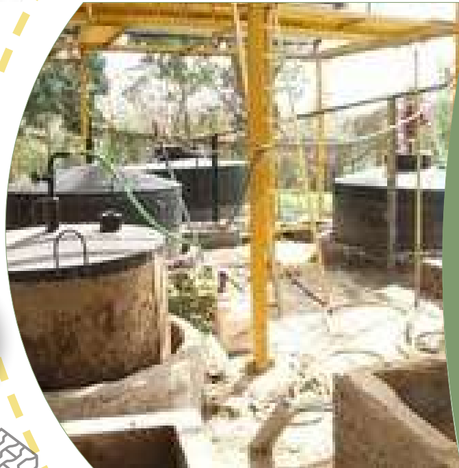
Image showcasing GEV Biogas plant at site, used to convert all kitchen and landscape waste to bio gas for cooking, resulting in zero waste site
