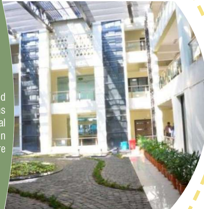
Central Atrium with louvers to provide shading & the courtyard above is misted to maintain thermal comfort
