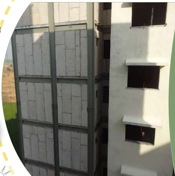
Photograph showcasing EPS cement sandwich panels for construction
