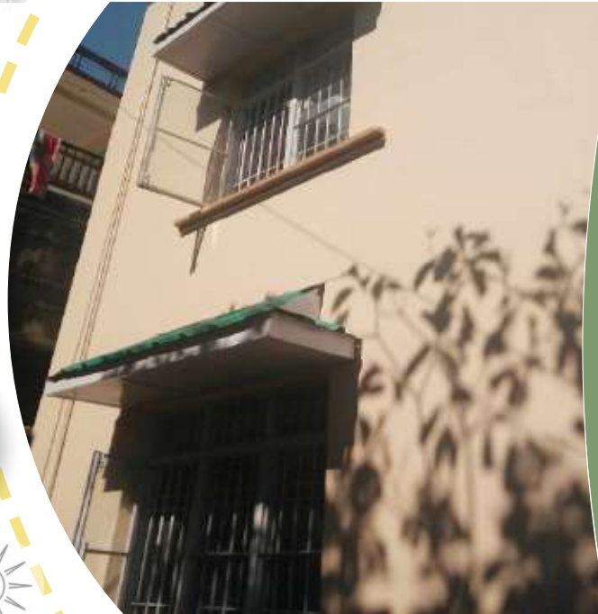
Image showcasing horizontal shading of windows on facade
