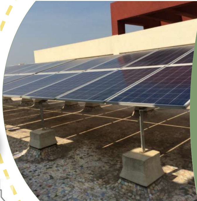
Image illustrating a rooftop with high Solar Reflectance Index (SRI) tiles, effectively reducing heat absorption, while solar panels provide additional shading and generate renewable energy
