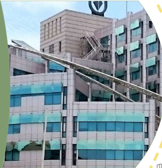
Close up image of facade of building showcasing shading of glazing
