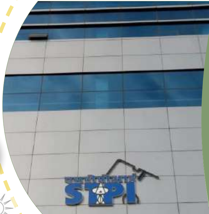
Image showcasing high-reflective DGU glass used for external glazing, effectively reducing heat gain and improving energy efficiency
