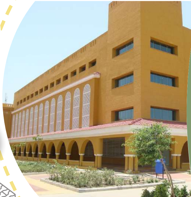
Image showing external façade of the building with shaded walkways along the edge of the building & extensive jalis to provide shade to windows
