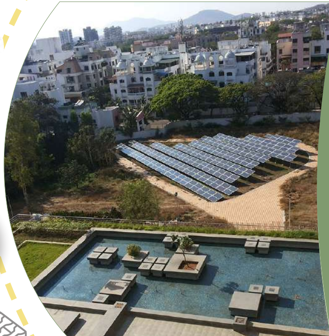
Image showcasing the terrace garden on the east side, shaded by PV panels and complemented by a water body for evaporative cooling Source: Landmark Design Group
