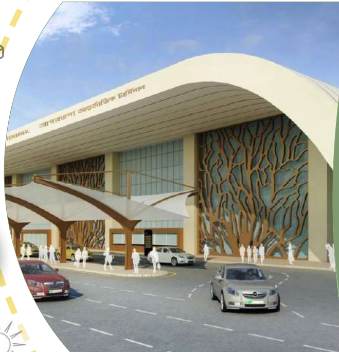
Rendered image showcasing extensive shading on the east-facing front façade
