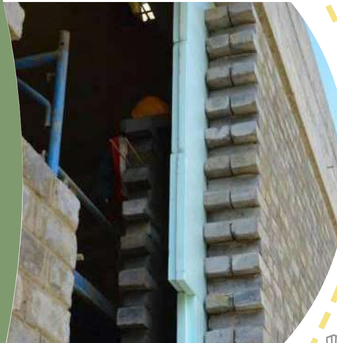
Image showing envelope construction with insulation & flyash brick
