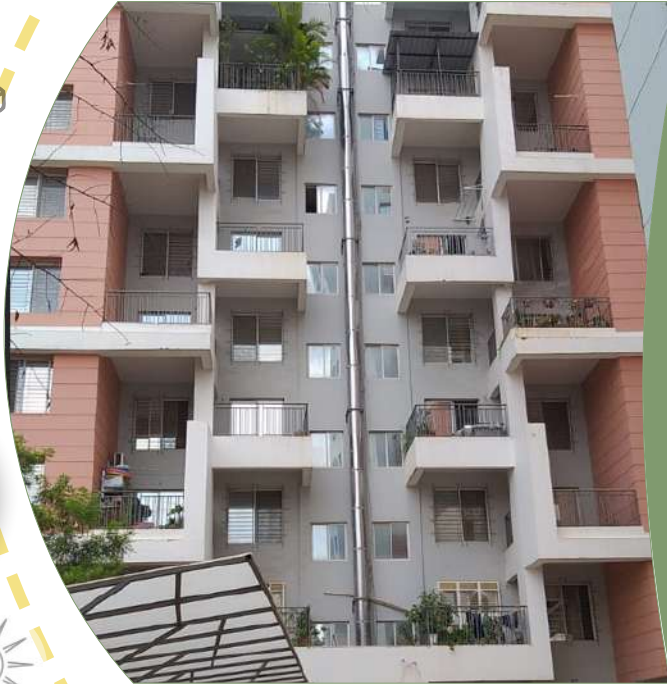
Image showcasing inset windows and strategically designed shading balconies that minimize heat gain while enhancing natural ventilation
