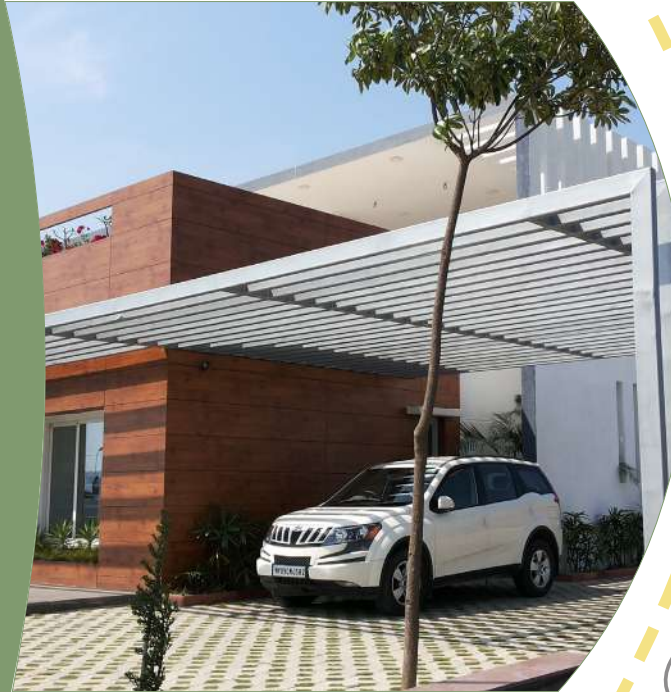
Image showing grass pavers used on site & pergolas placed for shading
