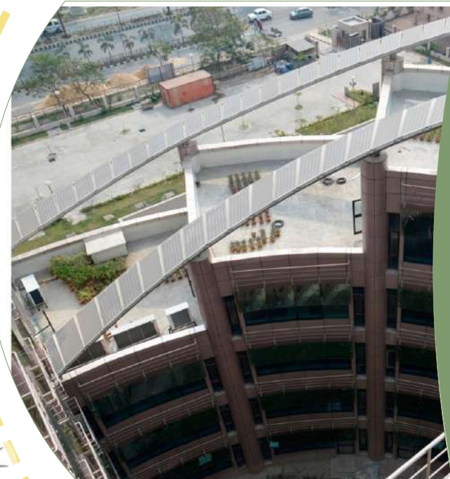
Image of the building showcasing BIPV along the stepped levels
