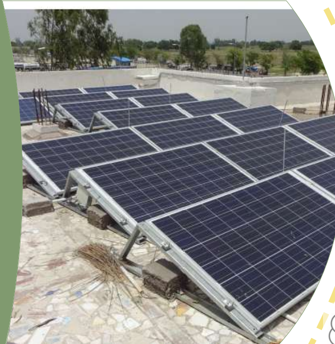
Image showing roof placed with high SRI tiles mosaic to reduce heat gain & solar panels
