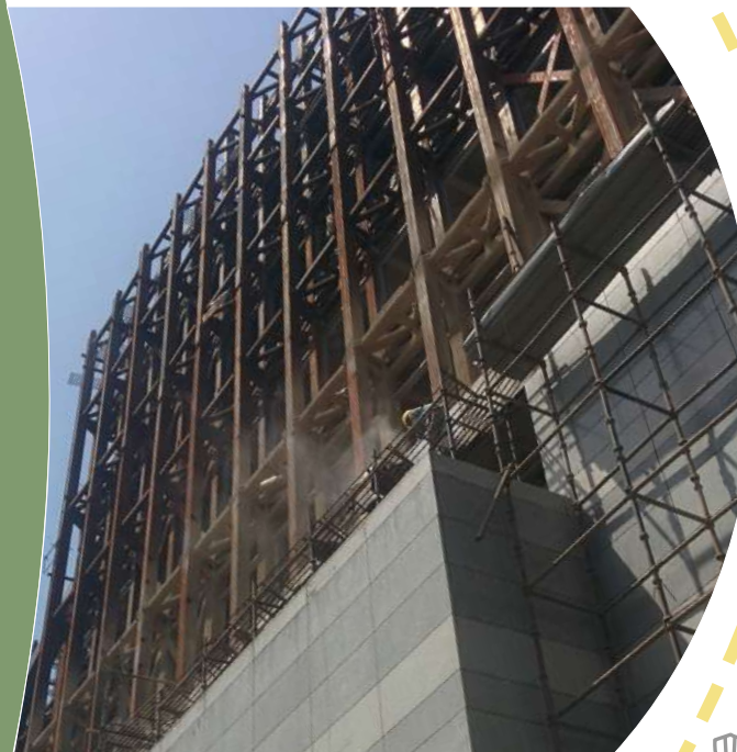
Image of facade under construction showing the steel framework constructed to reduce RCC structure
