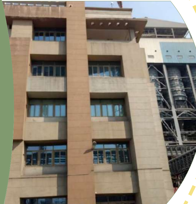
Close-up image of the façade highlighting window shading and self-shading achieved through varied building levels
