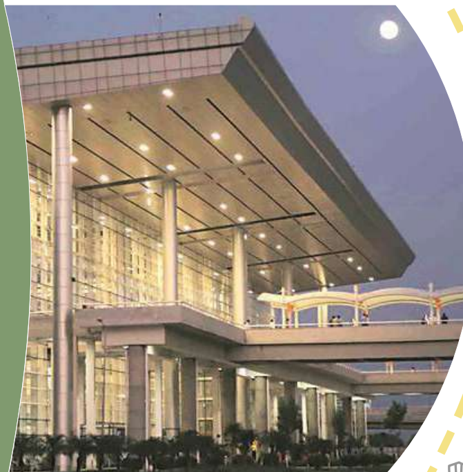
A close up image of the front facade of building showing the deep overhang in the project shading the façade
