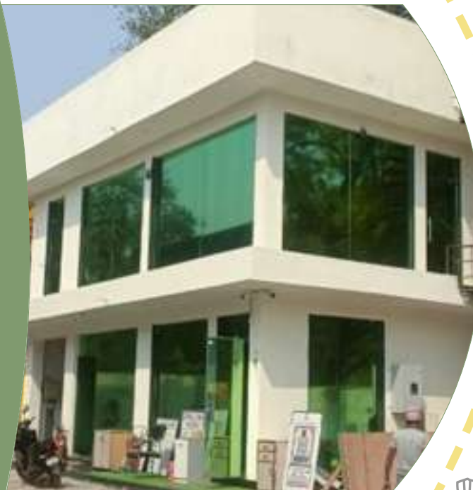
Close up image of facade of building showcasing use of tinted selective film on glass and shading in glazing
