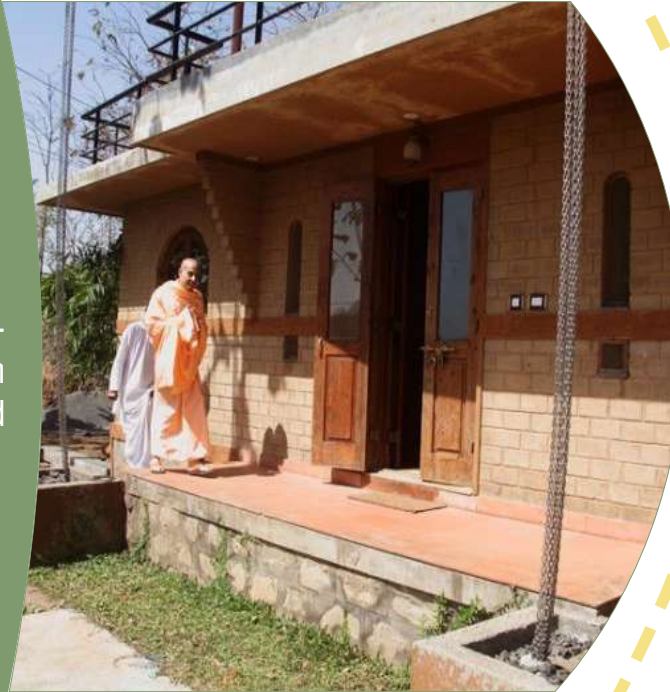
Image highlighting natural building materials, featuring a rain chain that directs water from the roof to a sump for efficient rainwater management
