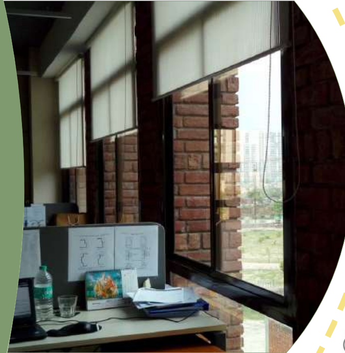
Image showing vertical fins for shading windows & natural light in the office space.
