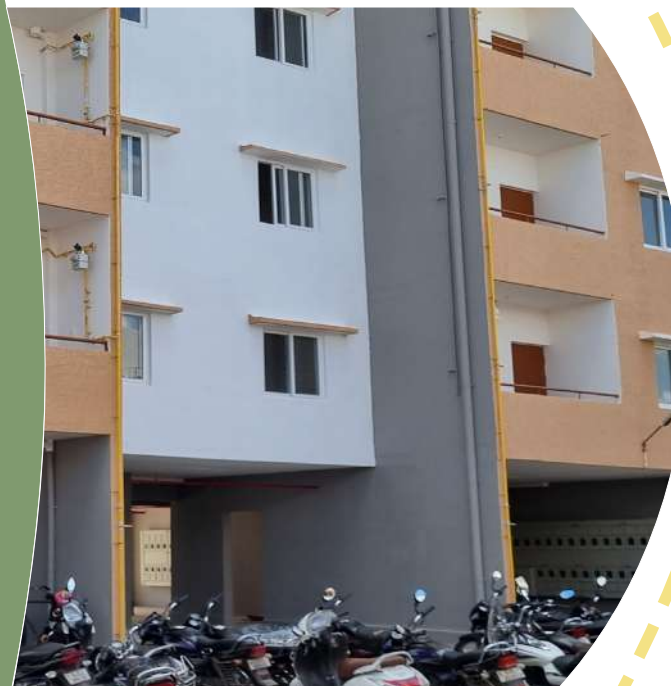
Photograph showing light coloured exterior with shading used for windows.
